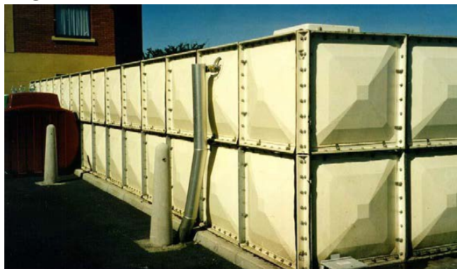
15150 x 4140 x 2000mm 120,000 litre (26,000 gallons) sectional water tank insulated to Format 30. Installed 1998.
