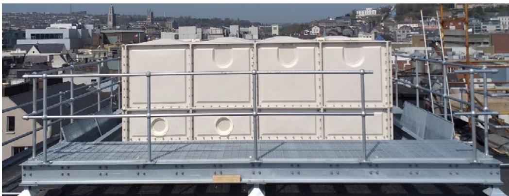
4150 x 4150 x 1500mm 24,000 Litre water tank insulated to F30
